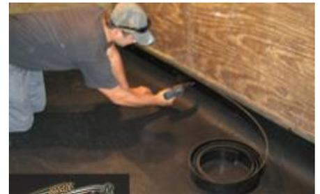
11. Once Enviroskin is completely secured along the stall, cut excess from above the baseplate.
