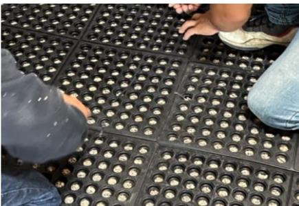
7. Secure the Enviromats together with the industrial strength cable ties using at least two per side. The last row of the Enviromats may need to be cut to fit along the edges of the stall. Do not allow the Enviromats to go up the walls of the stall. Cut the excess from the cable ties and push the connection below the anti-fatigue mat line.
