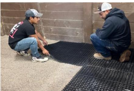
6. Facing into the stall, start in the front right corner. Set an Enviromat anti-fatigue mat on the Envirolyte with the two smooth edges of the Enviromat pressed into the corner against the stall walls. Keeping the smooth edge along the wall, snap the Enviromats.
