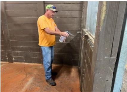
1. If installing Envirostall in an existing stall, spray stall walls with one-half gallon of Envirostall Smart Touch (based on a 12' by 12' stall). Use disinfectant at full strength. DO NOT mix disinfectant with water. New stalls do not need disinfected.
