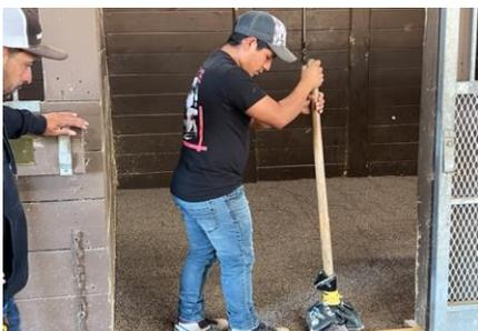
4. Use the tamper to tamp down the Envirolyte avoiding any build up or high spots, particularly in the corners. Using the level, again assure the Envirolyte is level.
