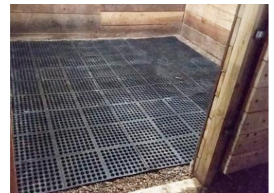
Cushioned mat laid over the storage aggregate.
